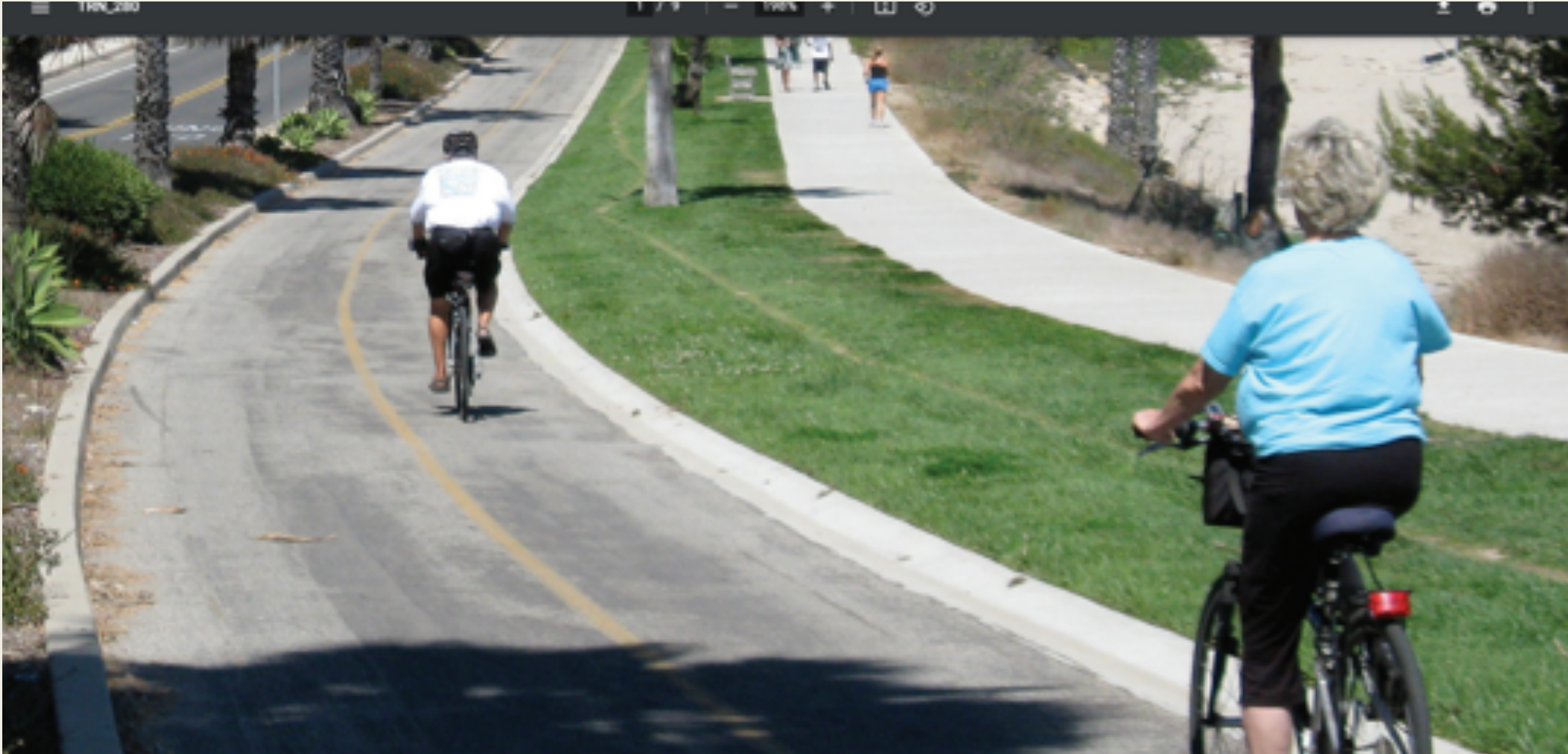
Example of Champlain RIGHTway (left), separate bikeway and sidewalk (right)—Santa Barbara, CA
